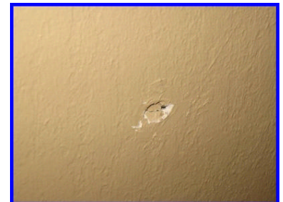
Wall damaged from door knob
