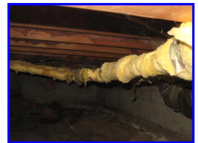
Piping not supported over 20 feet
