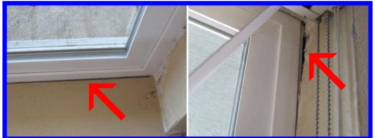
Caulking around windows is incomplete
