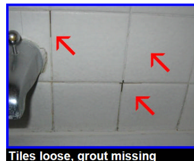
Tiles loose, grout missing
