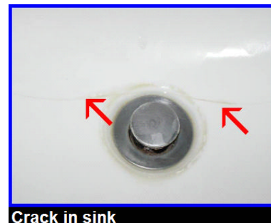
Crack in sink
