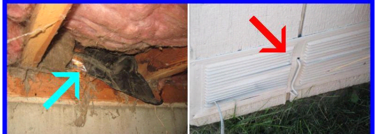
Vents closed and plugged
